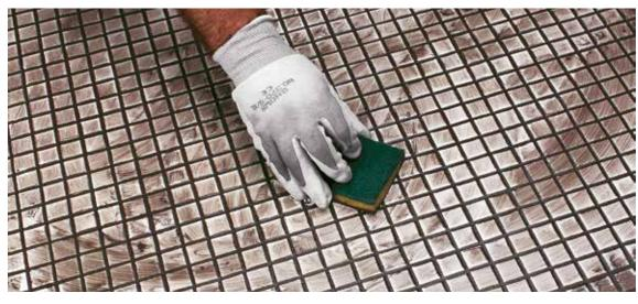
**TECHNICAL FEATURES:** Special flexible grout with rapid setting, for joints from 2 to 12 mm in wide. DEKOGROUT 2/12 grouts are composed of special cements, aggregates with a choice of granulometry and additives, it was designed to harden rapidly with minimum shrinkage to provide elevated mechanical resistance, good flexibility and minimum water absorption united with an attractive aesthetic appearance. They are available in various colors.
