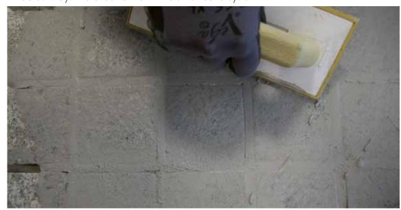
**TECHNICAL FEATURES:** Special flexible grout, rapid setting, for joints from 3 - 30 mm wide. The grouts DEKOGROUT-HF 1/30 are composed by special cements, aggregates with selected granulometry and additives and they are studied to harden quickly and with minimum shrinkage, until they develop high mechanical resistance, good flexibility and minimum water absorption, as well as pleasant aesthetic effect.
