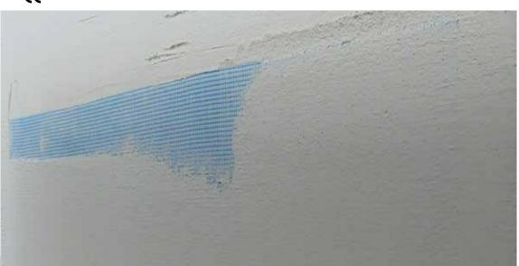
**TECHNICAL FEATURES:** BENFERPLASTER-07 WHITE is an adhesive/levelling mortar, fiber-reinforced for exterior insulation and finishing system, whose composition is cement, aggregates with selected grain size with diameter less of 0,7 mm, synthetic resins and special additives. Its formula has been created and developed to paste in a rapid and safe way all the boards used in exterior thermal insulation.
