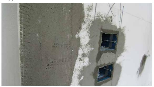
**TECHNICAL FEATURES:** BENFERPLASTER-07 GREY is an adhesive/levelling mortar, fiber-reinforced for exterior insulation and finishing system, whose composition is cement, aggregates with selected grain size with diameter less of 0,7 mm, synthetic resins and special additives. Its formula has been created and developed to paste in a rapid and safe way all the boards used in exterior thermal insulation.
