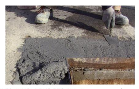
TECHNICAL FEATURES: BENFERCURE-VARIO-10 is a cementitious thixotropic mortar for the protection against corrosion of reinforcing steel, for concrete superficial protection conforming to:
