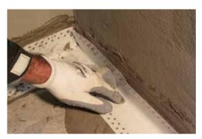
**TECHNICAL FEATURES:** ACQUASHIELD-2KF is a flexible elastomeric, 2-comp. polymer modified coating that waterproofs and protects concrete, masonry, brick and some natural stone substrates with crack-bridging properties. ACQUASHIELD-2KF has excellent adhesion characteristics and provides a seamless system which can be left as the finished surface\*, or can be top-coated with tiles, pavers, paint, or other coatings.
