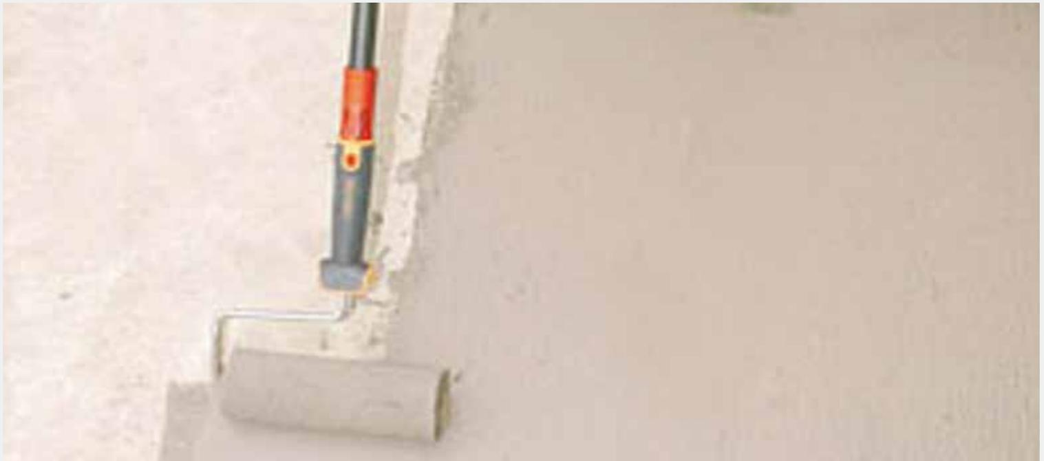
**Technical features:** ACQUASHIELD+ is a two-component mortar consisting of high resistance cements, fine aggregates with graded particle size (less than 0,3 mm), special additives (component A) and synthetic polymers in aqueous dispersion (component B).
