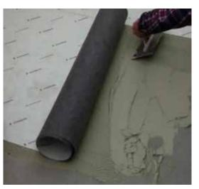
**TECHNICAL FEATURES:** MATADHESIVE is a thin-bed adhesive, for applications without voids in particular with profiled or large format tiles under time constraints.
