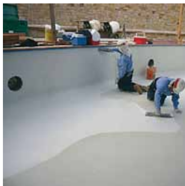
Trowel application under tiles
