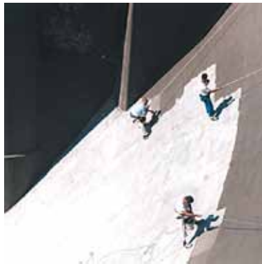
Brush application on a dam
