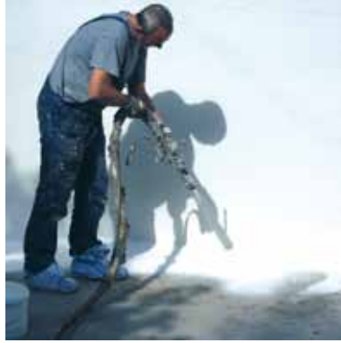
Spray application of a swimming pool
