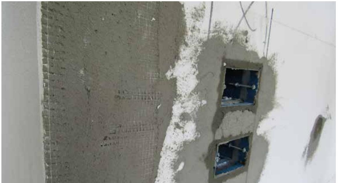
**TECHNICAL FEATURES:** BENERPLASTER-07 GREY is an adhesive/levelling mortar, fiber-reinforced for exterior insulation and finishing system, whose composition is cement, aggregates with selected grain size with diameter less of 0,7 mm, synthetic resins and special additives. Its formula has been created and developed to paste in a rapid and safe way all the boards used in exterior thermal insulation.
