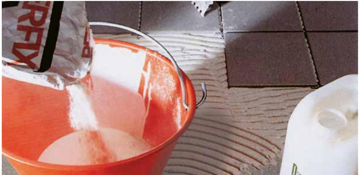
**TECHNICAL FEATURES:** BENFERFIX EXTRA is a cement based adhesive in white or grey with excellent workability and grip, for the interior and exterior application of ceramic floor and wall coverings. Its formula is the result of years of experience and guaranteed by thousands of applications in Italy and abroad, each year.
