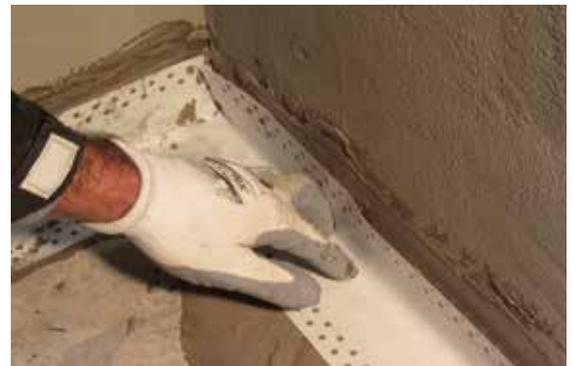
**TECHNICAL FEATURES:** ACQUASHIELD-2KF is a flexible elastomeric, 2-comp. polymer modified coating that waterproofs and protects concrete, masonry, brick and some natural stone substrates with crack-bridging properties. ACQUASHIELD-2KF has excellent adhesion characteristics and provides a seamless system which can be left as the finished surface\*, or can be top-coated with tiles, pavers, paint, or other coatings.
